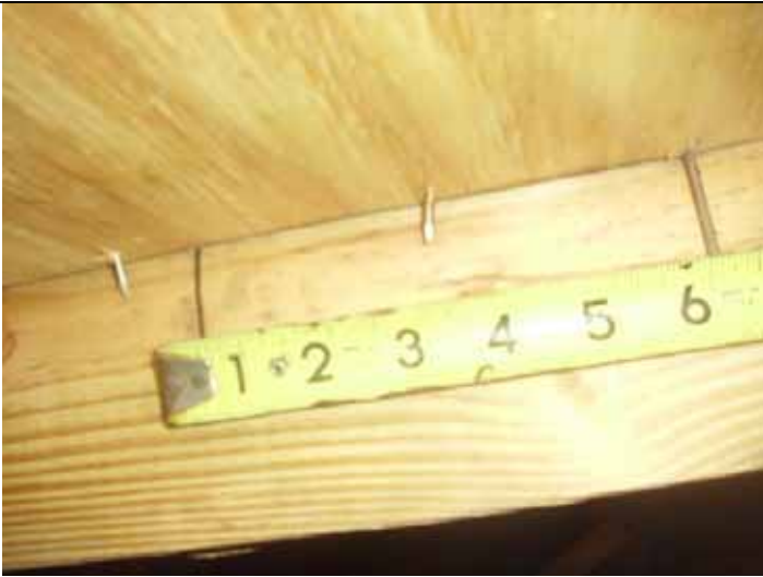
Roof deck attachment
