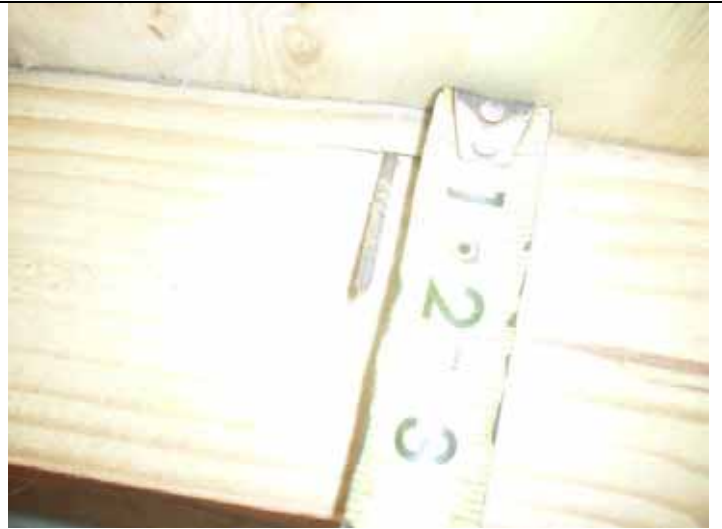
Roof deck attachment
