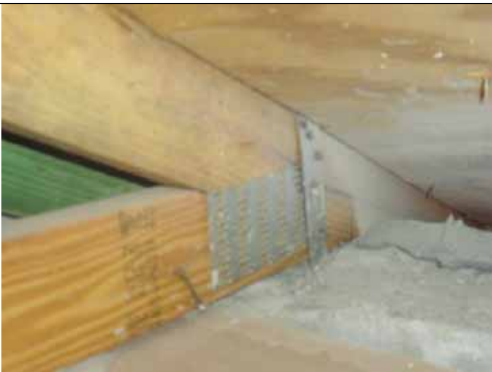
Roof to wall attachment
