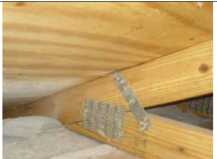
Roof to wall attachment
